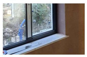
Take extra care during building phase of property. Plaster, cement and building dust will attack and corrode the hardware.
